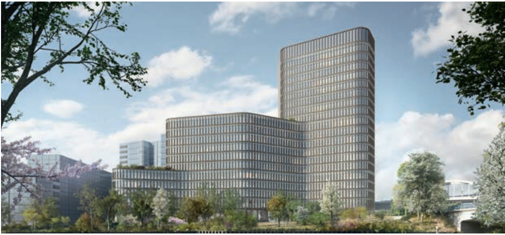
UPBEAT Berlin ----- Project under construction
