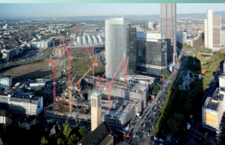
CONSTRUCTION SITE TOWER 185 CITY DISTRICT EUROPAVIERTEL, FRANKFURT
