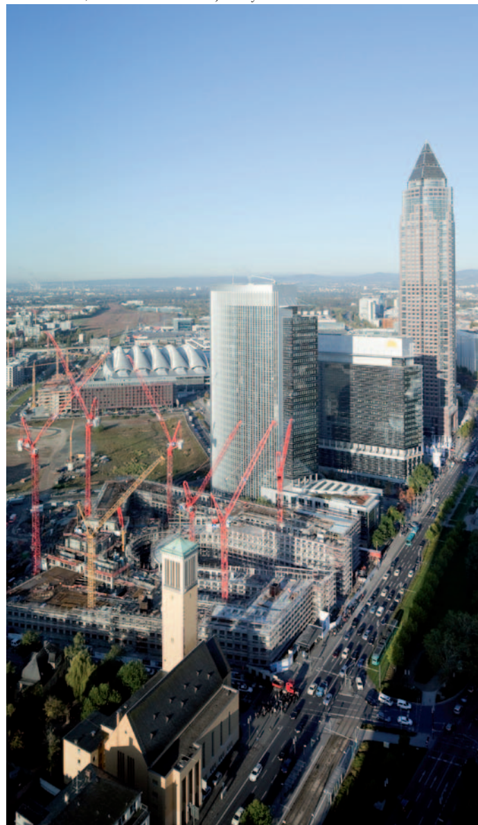
TOWER 185 Frankfurt, construction site as of January 2010
