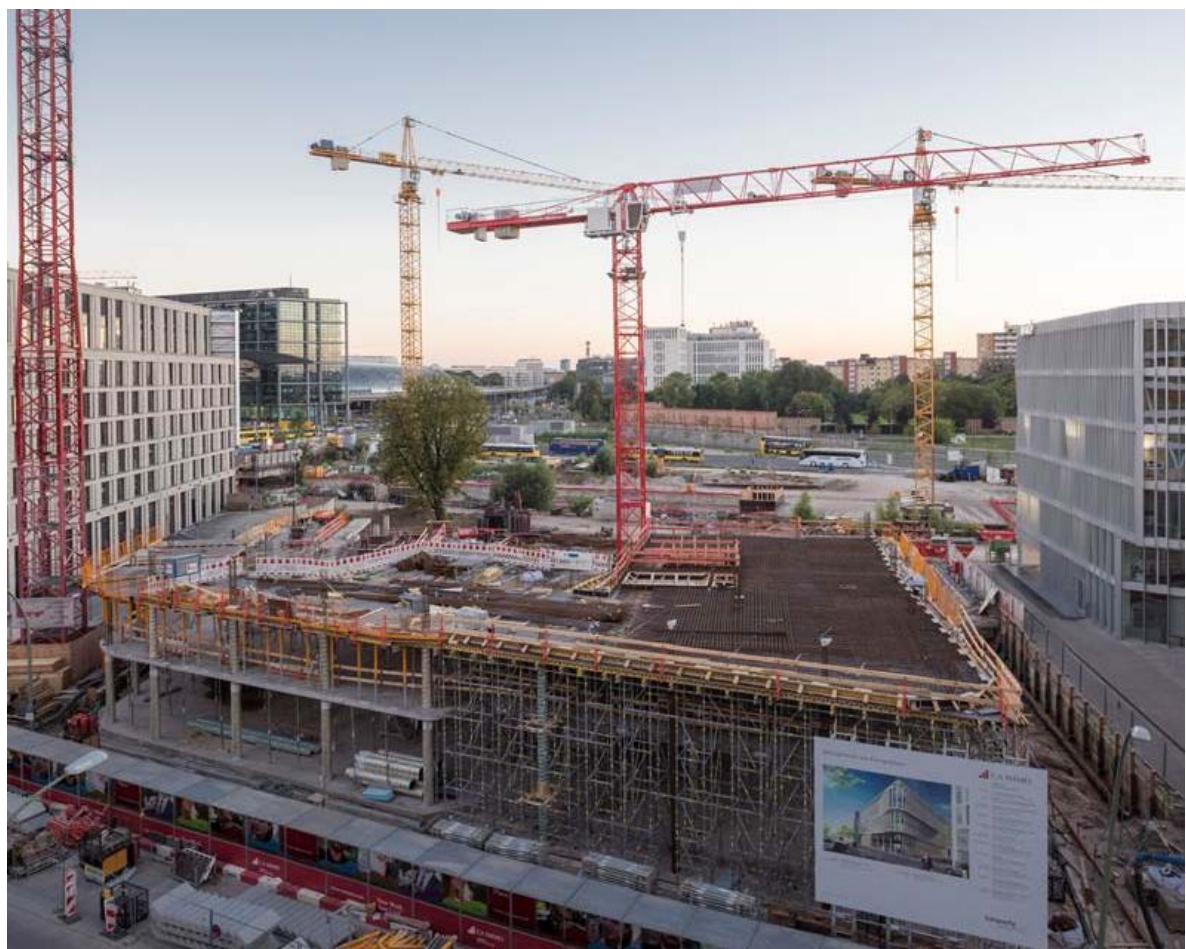
Under construction: KPMG building in Berlin
