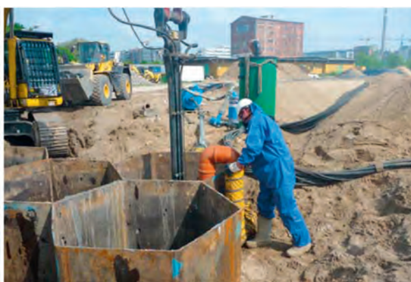
Preparing the ground: Site development by specialist construction subsidiary omniCon in Berlin's Europacity
