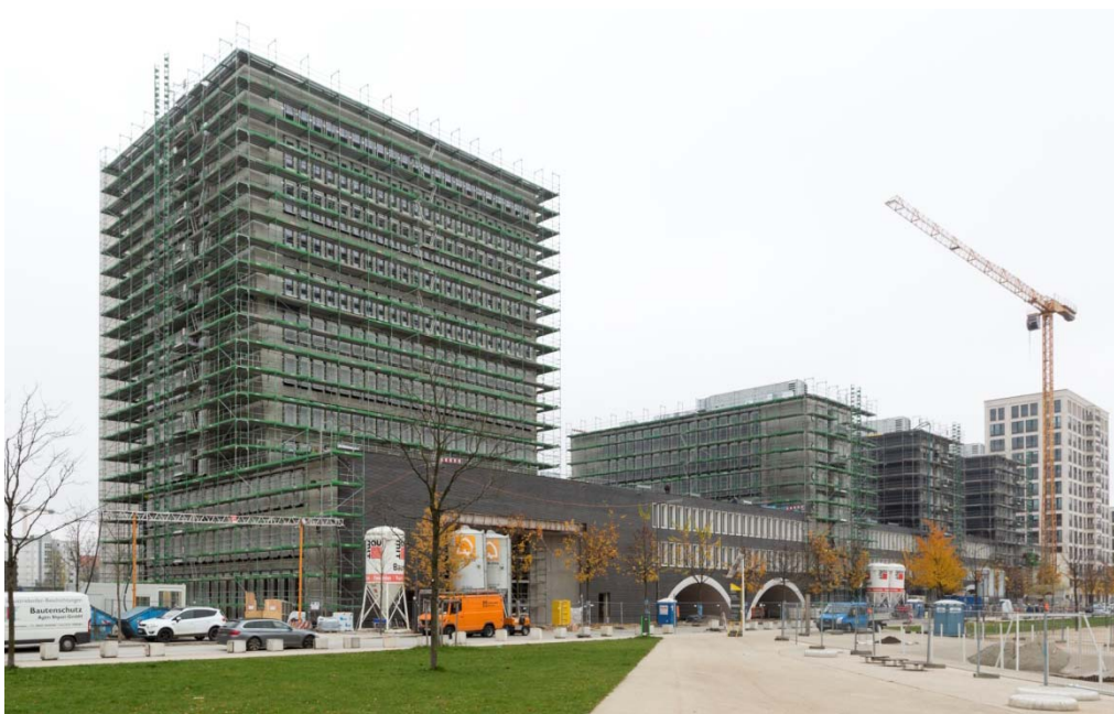
Construction site of the Kontorhaus office building in Munich
