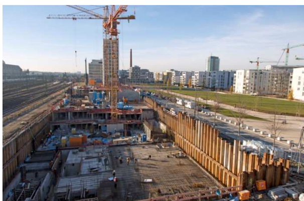
Construction site of Kontorhaus in the Munich Arnulfpark
