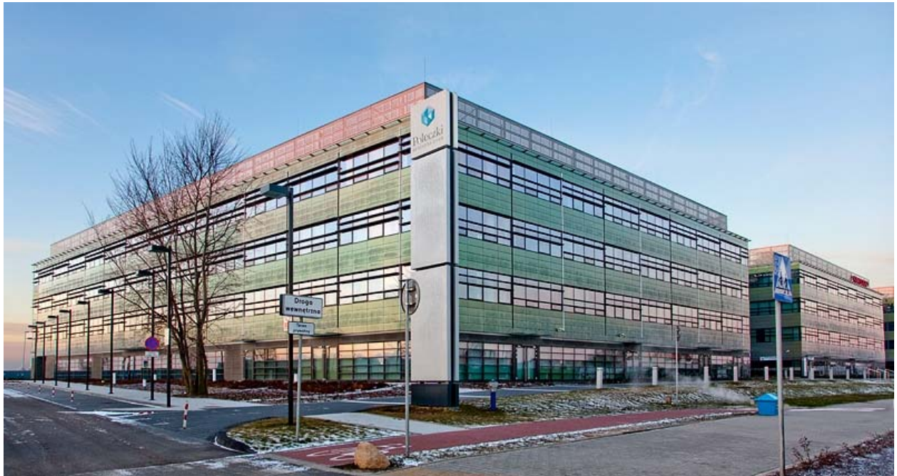
Poleczki Business Park, Poland, construction phase 1
