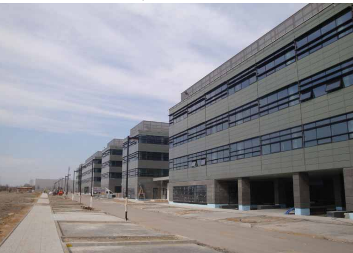
POLECZKI BUSINESS PARK Warsaw, Phase I finished
