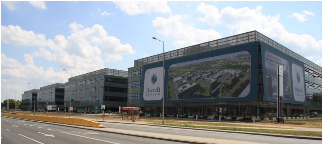
WARSAW, Poleczki Business Park, construction phase 1
