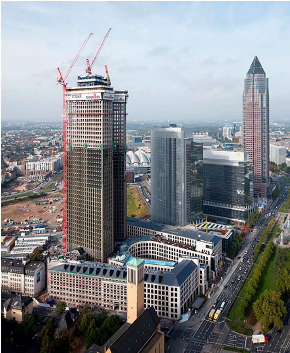
FRANKFURT, construction site of Tower 185
